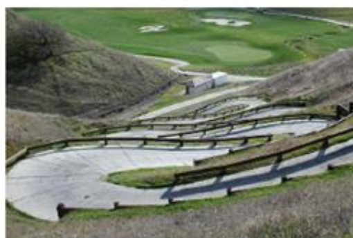
A “switchback” route
