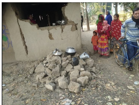
Figure No. 6 Hut Damage by elephants
